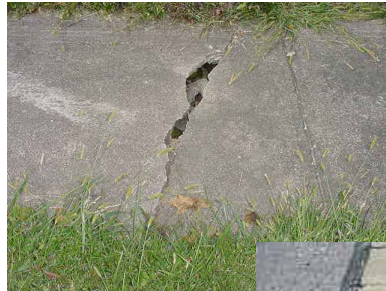
ANY SIDEWALK BLOCK (BASED ON 20 SQ. FT.) HAVING A CRACK OR CRACKS IN IT OF AT LEAST 1/2 INCH WIDE WITH A MINIMUM OF 4 LINEAR FEET IN ONE BLOCK. (VARIOUS SIZE BLOCKS WILL BE EVALUATED PROPORTIONALLY.)
