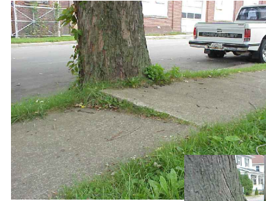
BLOCKS, OR PORTION OF BLOCKS, THAT CAUSE AN ABRUPT CHANGE OF 1 INCH PER FOOT (OR MORE) IN ANY DIRECTION OF THE SIDEWALK.
