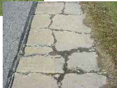
ANY SIDEWALK BLOCK (BASED ON 20 SQ. FT.) HAVING A CRACK OR CRACKS IN IT OF AT LEAST 1/2 INCH WIDE WITH A MINIMUM OF 4 LINEAR FEET IN ONE BLOCK. (VARIOUS SIZE BLOCKS WILL BE EVALUATED PROPORTIONALLY.)
