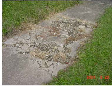
ANY SIDEWALK THAT IS DETERIORATED OR SHOWS SURFACE SPALLING, LEAVING IT VERY ROUGH, UNSAFE, OR WITH AGGREGATE PROTRUDING.
