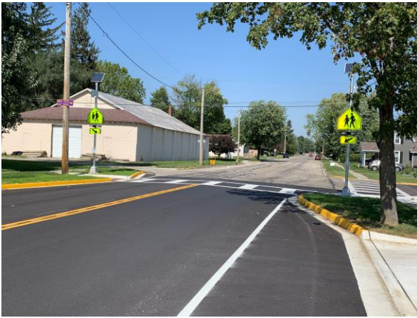
Curb Bump out – East School, Aukerman St.
