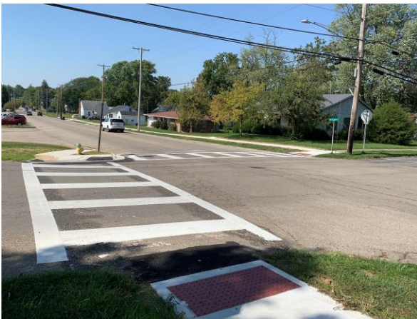
Intersect Maple & St. Clair - ADA Ramps
