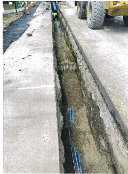
Installing Water Line North Barron Street
