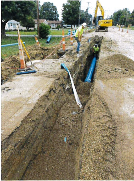
Installing Water Line North Barron Street
