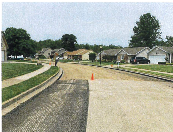
Washington Landing - Milling
